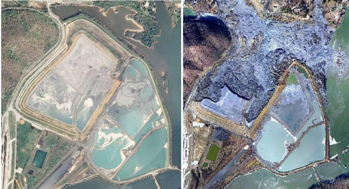
Figure 1: Aerial photographs comparing the Kingston Fossil Plant ash disposal area before and after the massive slope failure on December 22, 2008.
